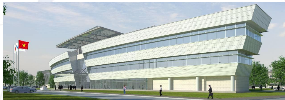
Management Center and S/C Control Center
