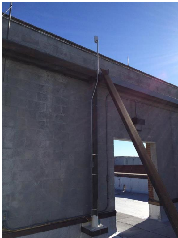
SKYCAM1 at GSFC Building 33 Maryland, USA
